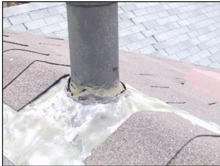
2. Stack flashing should be sealed.
