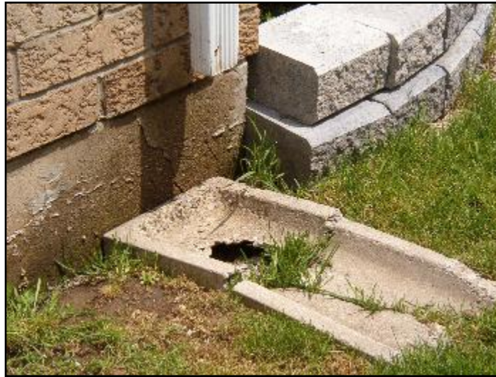
3. Downspout should be extended away from home
