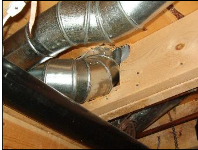
4. Double joist cut for ductwork
