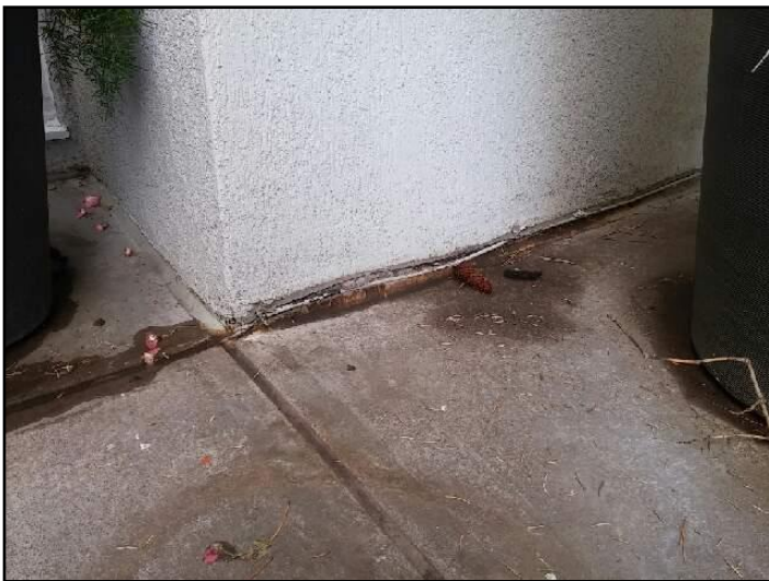
Too Close to Grade
