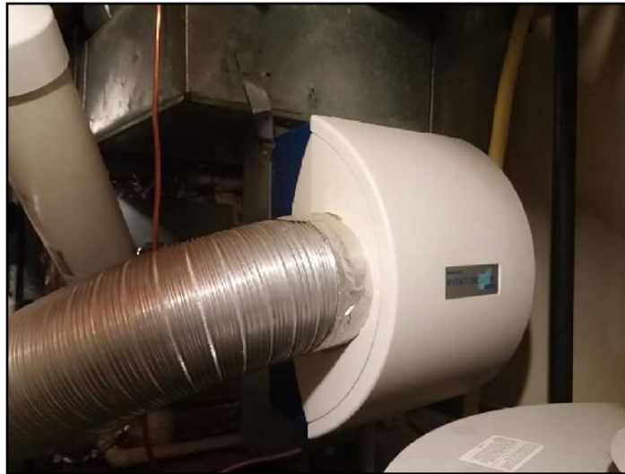
Whole House Humidifier - Second Floor
