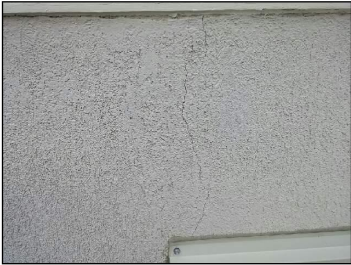
Cracks in Stucco
