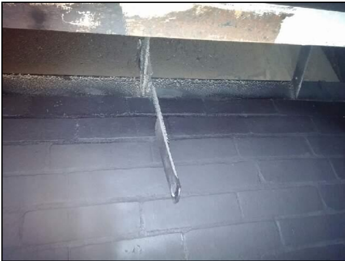
Damper Closed Position
