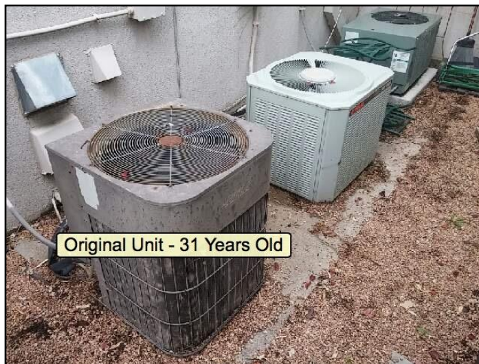
Lennox AC - Serves the Basement
