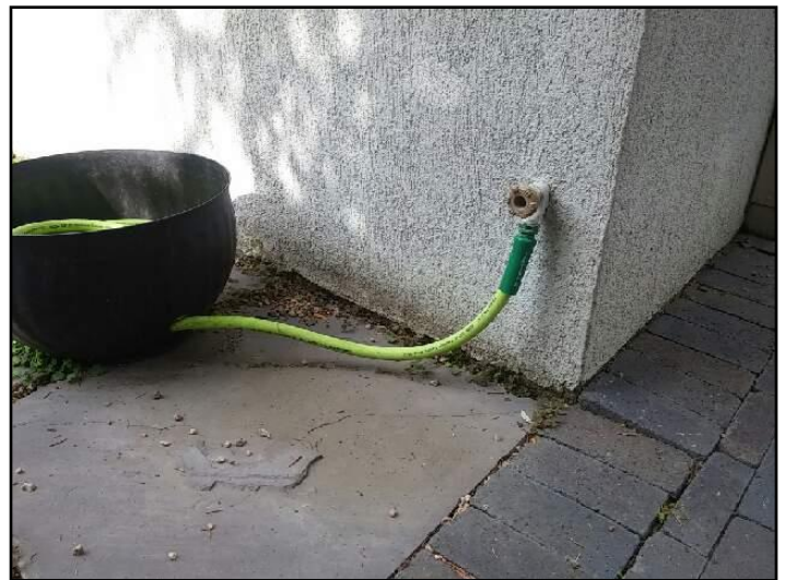
Too Close to Grade
