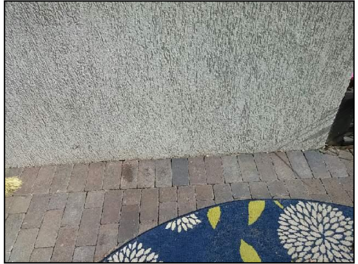
Stucco Below Rear Paver Patio
