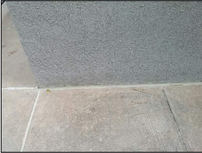
Sealed the Stucco at Front Patio
