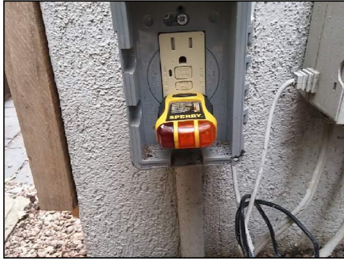
AC Service Outlet - East Exterior Wall
