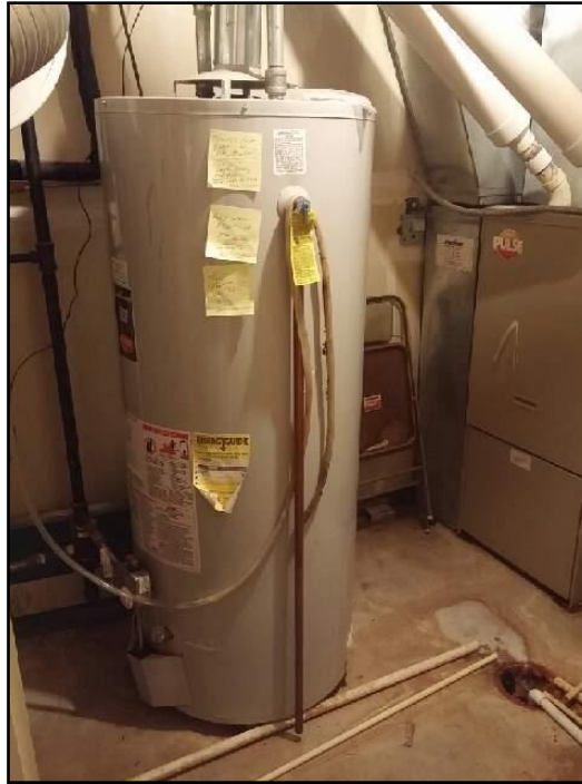
Water Heater - 15 Years Old
