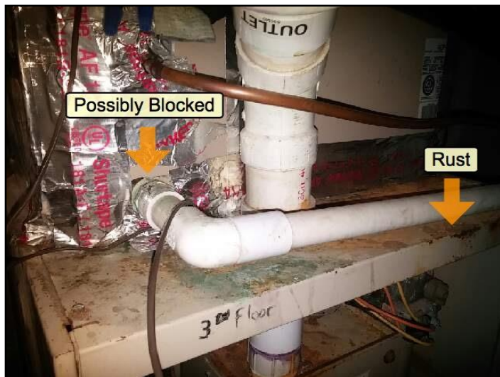
2nd Floor HVAC System
