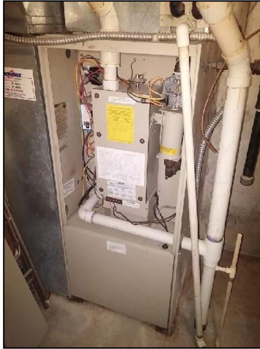
Main Floor Furnace
