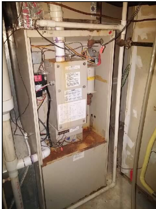
Second Floor Furnace
