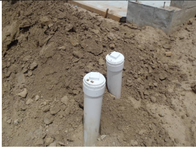
Sewer Clean Outs – South Exterior Garage
