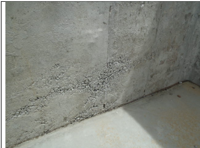
East Wall – Aggregate At Bottom of Wall
