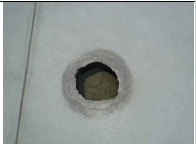
Pier Pads in Place – Column Attachment Sites
