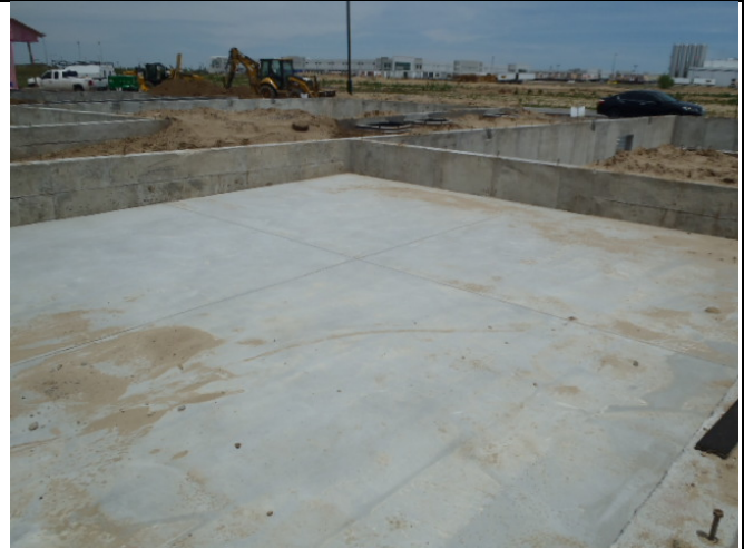
Garage Slab – Control Joints Cut In
