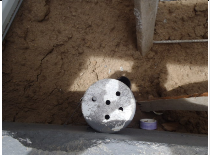
Window Well Drains – Each Basement Window
