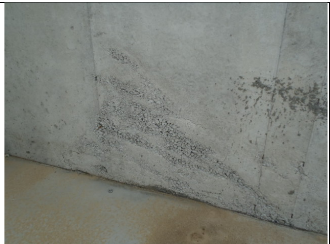
South Wall – Aggregate At Bottom of Wall
