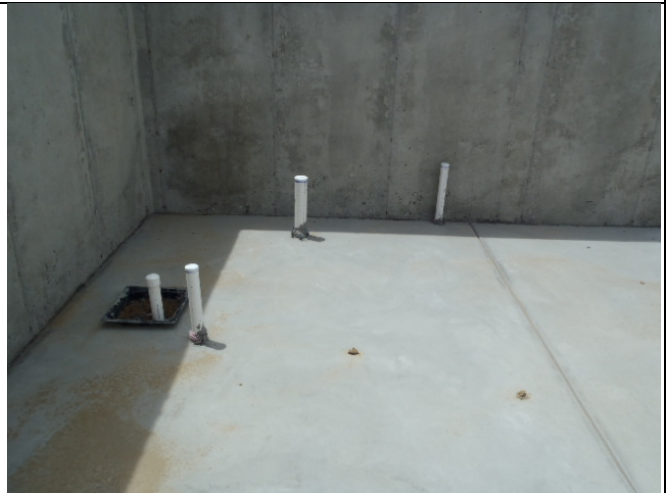
Roughed In Plumbing
