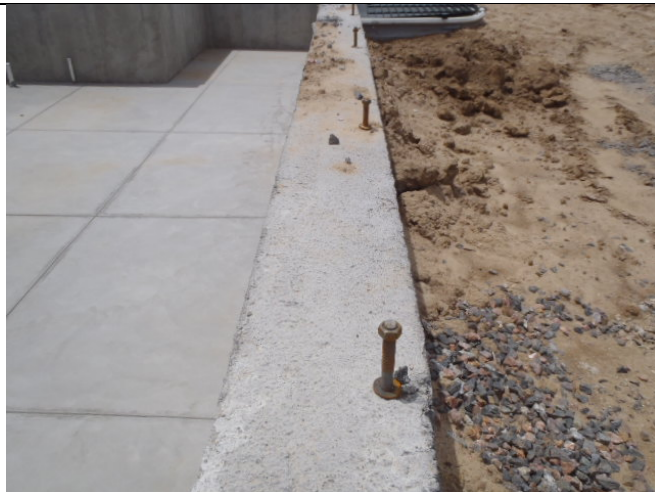
Anchor Bolts – Wall Attaches to these Bolts
