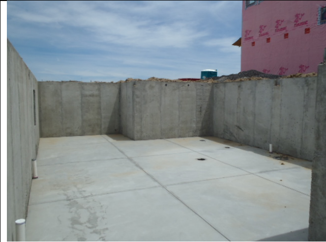
Basement Slab – Control Joints Cut In
