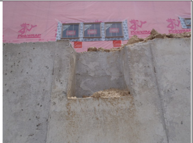
Beam Pockets – Cut Into Place
