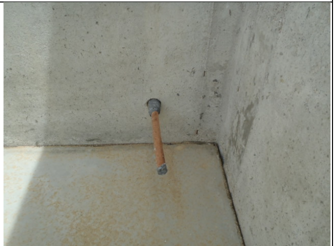
Main Water Line Plumbed – East Wall
