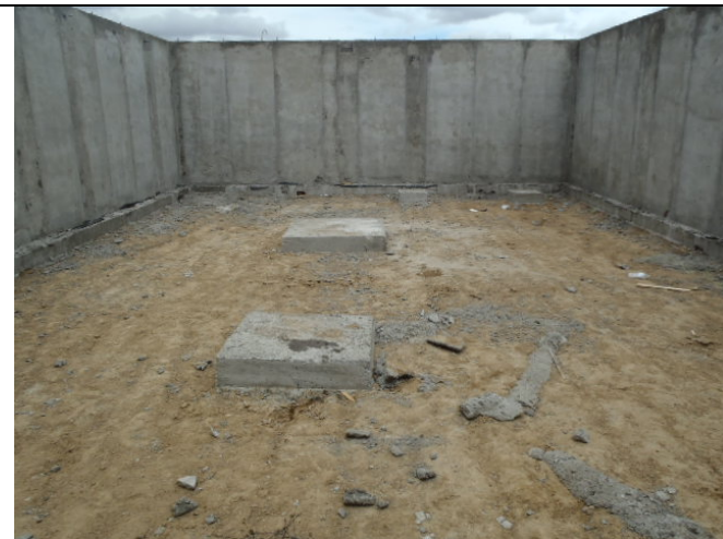
Pier Pad – Prior to Slab Being Poured
