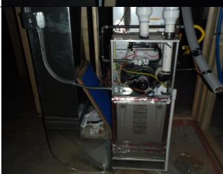
The furnace was installed with the AC coil in the basement. Installation of this system is appropriate. The system will be tested during the FINAL inspection.
