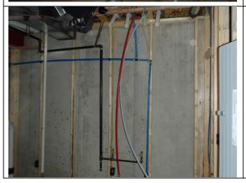
The home is plumbed for a tankless water heater in the basement. All components are present, however the tank typically does not get installed until the home can be properly secured.
