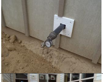
The main gas line inside the home has been installed. The builder is waiting on Xcel contractors to install the meter itself. Once that occurs a pressure test will occur. The pressure gauge is installed for the pressure test.
