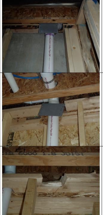
There was a plumbing nail plate on the North wall of the basement bedroom that was not of proper size, see photo.
