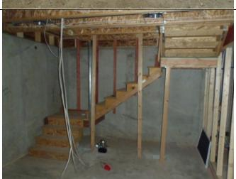
There were 2x4 temporary posts placed under the basement staircase. Two steel columns will replace these temporary posts to ensure longterm stability.
