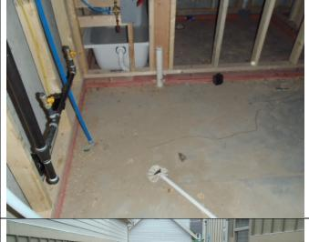
The basement floor drain had a vent present, however an air admittance (studor) vent was not installed. This usually occurs prior to the City's FINAL plumbing inspection.
