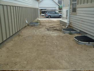
The grading around the proper is not to FINAL grade as of yet. This occurs at the final stages of the home building process. It is imperative that we have lot slope that moves away from the home's foundation.
