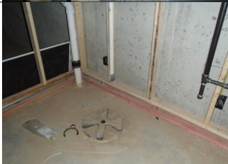
The sump pit had a discharge pipe to the exterior installed at the time of the inspection. This is an indication that a pump will be installed in the pit.
