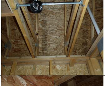
Soffit baffles are NOT in place to prevent insulation from blocking the soffit vents when the insulation is installed. These baffles are typically installed prior to the drywall installation.
