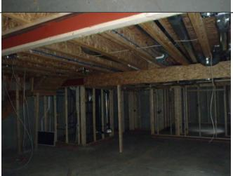
This pictures shows the temporary wood post supporting the steel column in the basement.
