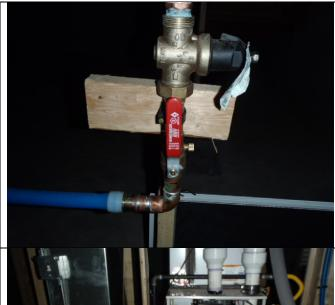
The main water shut-off valve is located on the East wall of the basement mechanical room. There is also a main water shut-off valve on the East wall of the basement living room.
