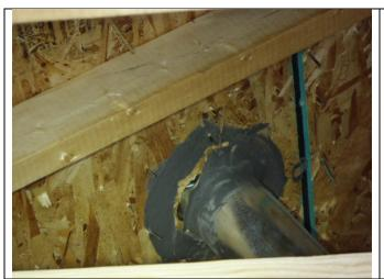
The laundry room vent fan duct, where it terminates to the exterior through the roof, had mastic that was damaged.
