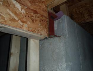
The steel beams in the basement had not been grouted into place at the time of the inspection. This usually occurs once the framing is in place and the City has conducted their framing inspection.
