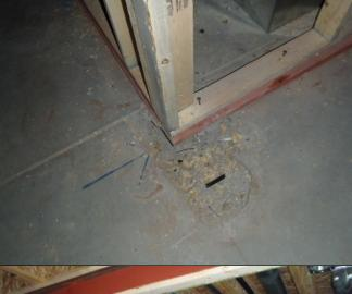
There was a pier in the basement that appeared to be covered and then uncovered. This pier is used to secure a steel column to support the steel I-beam above. However, it appears that the wall assembly for the basement mechanical room was built over the top of this pier.
