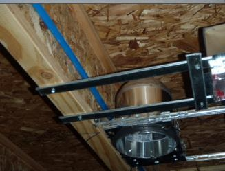
There was a water line that ran too close to a can light fixture in the basement living room ceiling.
