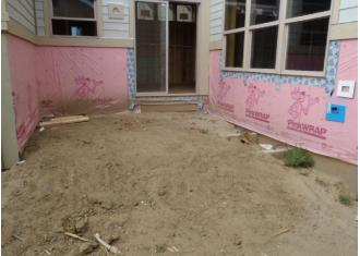
The rear patio has not been poured. Before they pour this concrete patio, metal flashing will be installed around the perimeter of the exterior walls to prevent the walls from becoming damaged from the moisture content within concrete.
