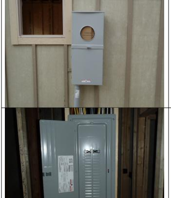
The main electrical panels and disconnects are located on the South exterior garage wall.
